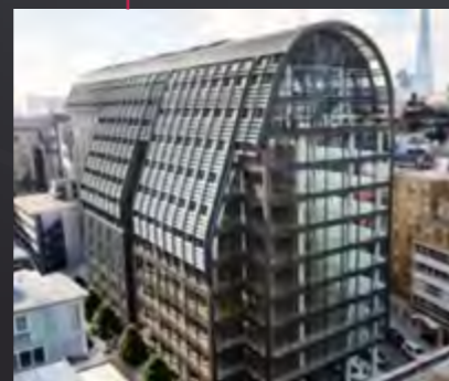
LUMINARY LONDON, ROMAN WALL Developer: Urban Nest Scheme: 650 student beds, 10,000 sq ft incubator space for Kings College alumni and 49,000 sq ft offices Status: Completed 2022
