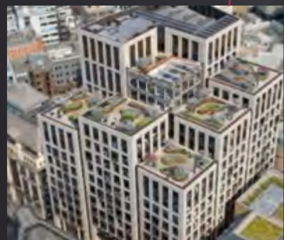
80 FENCHURCH STREET Developer: Partners Group Scheme: 250,000 sq ft Grade A offices Majority pre-let to Arcadis and Royal London Status: Completed Q1 2021
