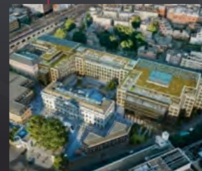
ROYAL MINT COURT Developer: Embassy of the Peoples Republic of China Scheme: Planning consent for a 600,000 sq ft development including 2 acres of public realm. Acquired by China in 2018 to house its new London Embassy. Status: Further planning application submitted
